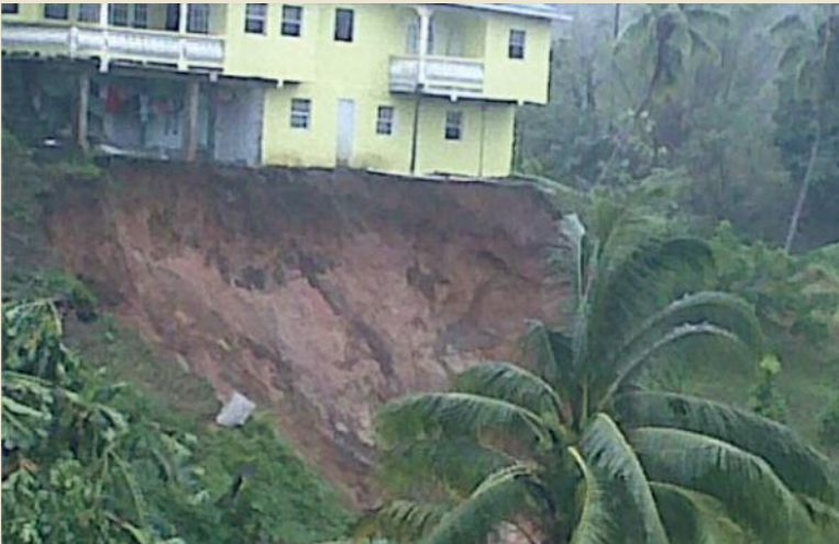
Hurricane Tomas damage in St Lucia
