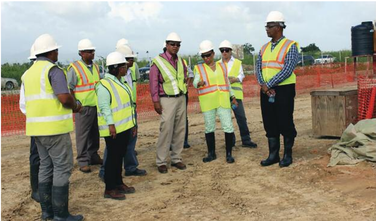
Principal V. Eudine Barriteau with the ACUITAS Engineering team at the development site in Chaguanas, Trinidad & Tobago. The construction of Phase 1 is off the ground with the focus being on draining and laying down underground infrastructure to support the Campus's buildings
